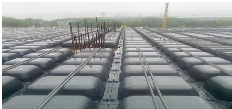
Figure 10- General view of slab formwork
